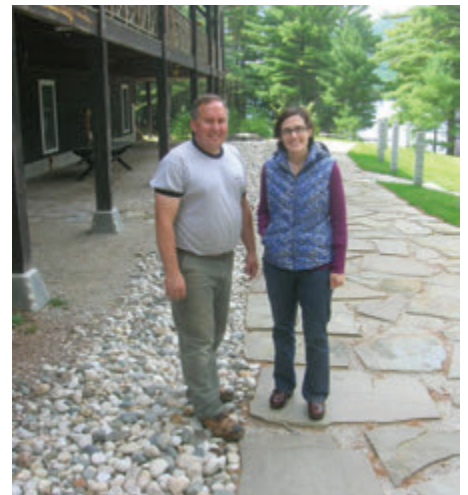
Spencer Ordway and Laura Ordway, directors at Winona Camps, stand on seven feet of crushed stone drip edge installed to catch roof runoff
