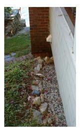
**Installation**: Dig a trench that is 18" wide and at least 8" deep along the drip line. Slope the bottom away from the house so that water will drain away from the foundation. Make sure to dispose of the soil in a flat area where it cannot be washed into the lake. Fill the trench with  $\frac{1}{2}$ " -1\frac{1}{2}" crushed stone. The front and sides of the trench may be edged with stone or with pressure-treated lumber to hold the stones in place.
